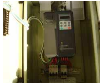
Figure 51: Special pump inverter for direct connection to solar system
