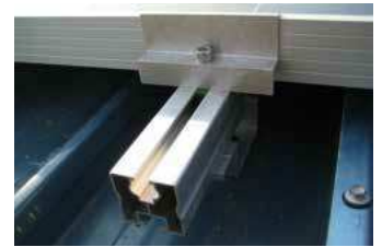
Figure 45: Standard module fasteners
