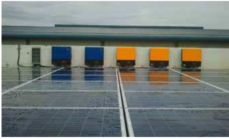
Figure 52: Standard grid inverters for grid or diesel generator connection
